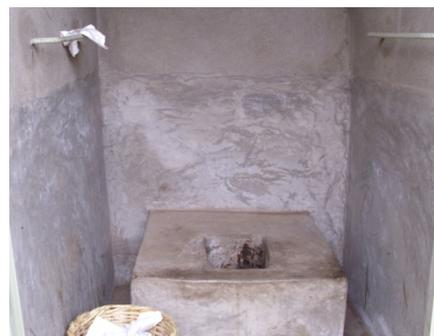
Figure 5. Raised toilet seat with handrails on side walls <sup>6</sup>
