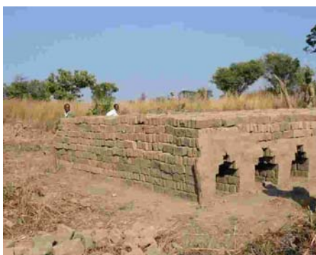
Making bricks for new classrooms
