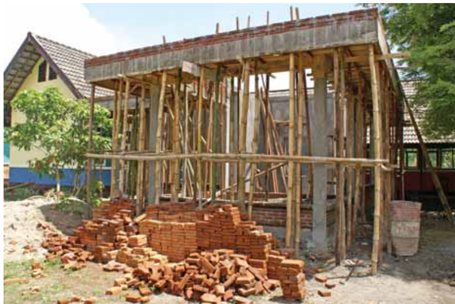
The new library under construction
