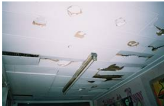
Photo by UK secondary school students of damaged school ceiling
