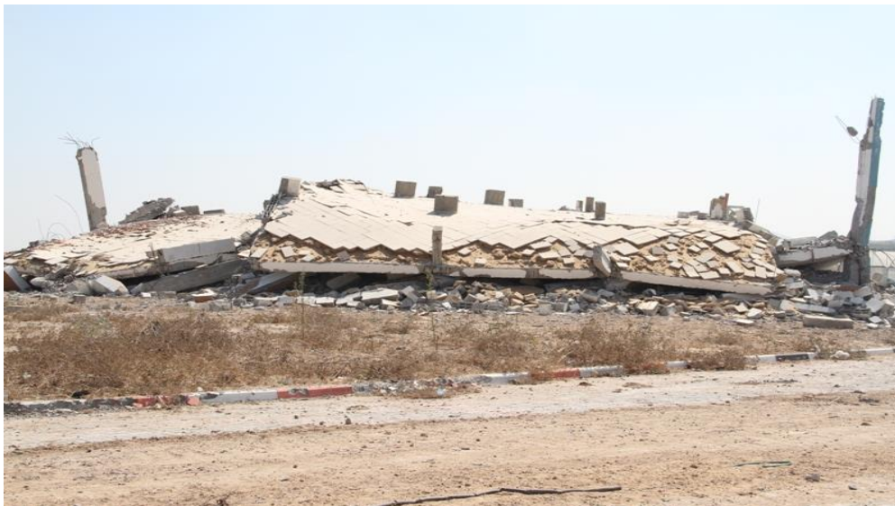
Image 6 Al Azhar University, Beit Hanoun, collapsed building © Alazhar University
